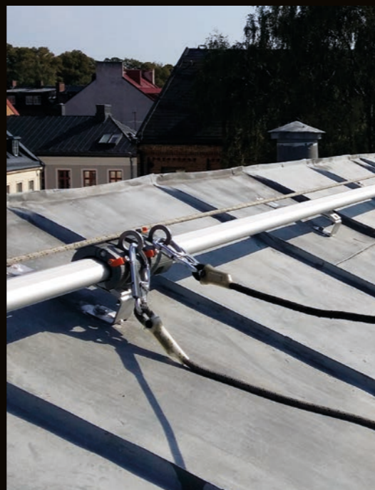
Boden-Montage | Floor installation
